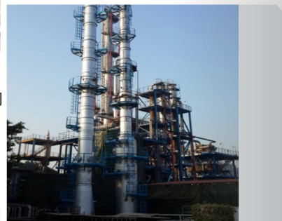
脱硫塔/Desulfurization Tower 规格/Specification: OD1200mm X 12mm X 16800mm
