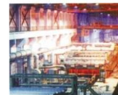
Annealing Furnace 46Meters Long
