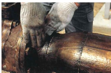
c. Application of PF Mastic
