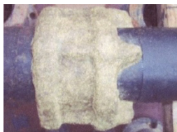
Filling with Mastic
