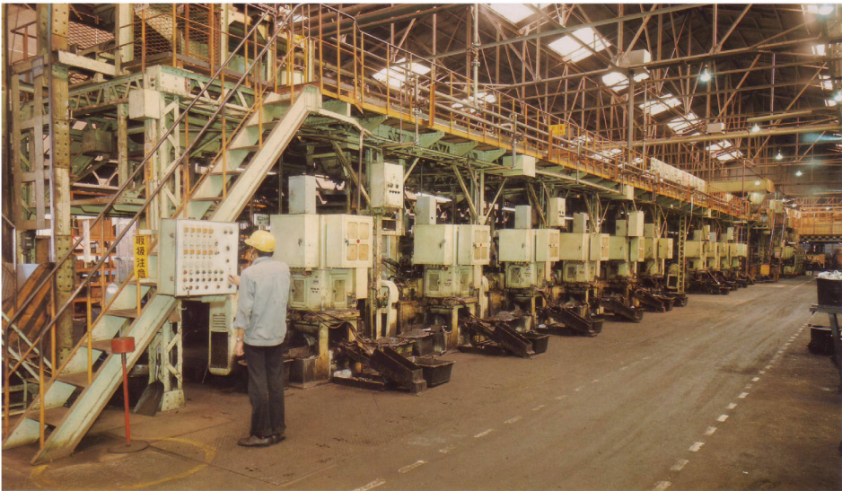
Modernized Tapping Shop
