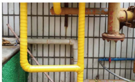
Corrosion prevention for tee & elbow
