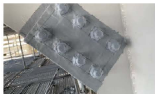
Corrosion prevention & sealing for bolt
