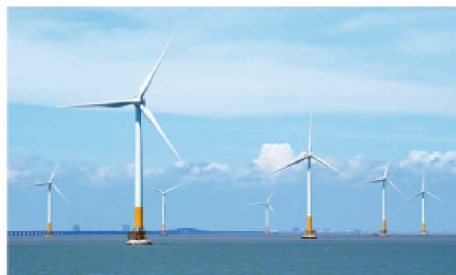
Corrosion prevention for offshore wind power
