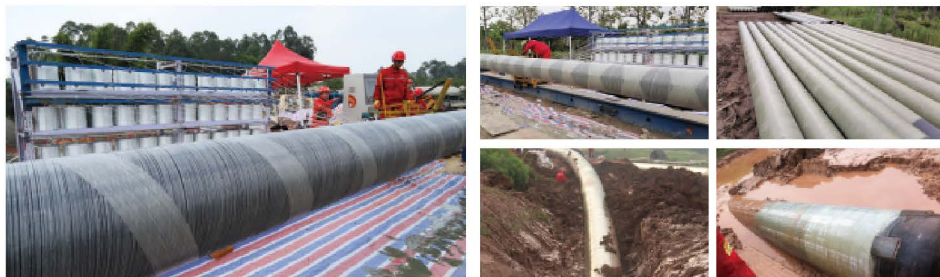
GFRP Mechanized Prefabrication Technology for Pipeline Directional Crossing By HDD
