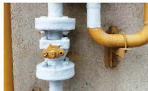
Corrosion prevention & sealing for flange
