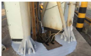
Corrosion prevention & sealing for steel structure
