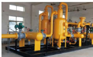
Corrosion prevention & sealing for oil & gas station
