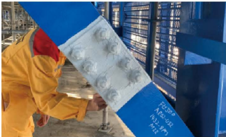
Bolts Corrosion Prevention In Formosa Plastic
