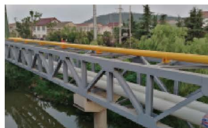
Corrosion prevention & sealing for outdoor pipelines
