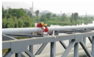
Corrosion prevention & sealing for steel pipelines.
