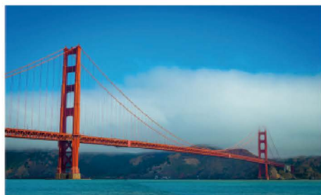
Corrosion prevention for bridge & vessel
